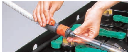
Start of water refilling: Opening the faucet automatically starts refilling water into all batteries (be sure to open the faucet fully).
